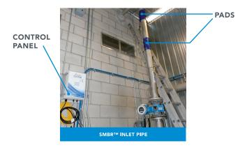
A short time after the beginning of trials, scale removal was confirmed by higher loads of TSS in the SMBRTM effluent. In addition, within 5 weeks of testing, a 70% decrease of the media's scale deposit was measured. The ELSC system provides a permanent solution to scale related maintenance costs, such as high pressure washing and chemical cleaning.
